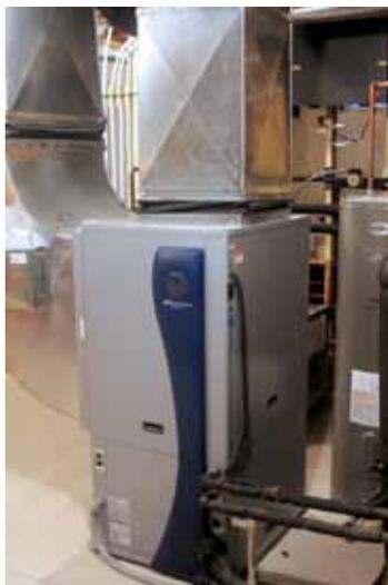
Pictured above is the WaterFurnace 5 Series water-to-air heat pump for cooling load and heating zones without radiant floor heat.
