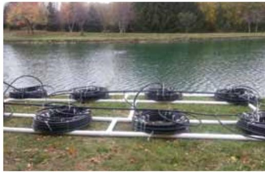
The geothermal loop system was installed in a pond. This is where the B&D flow center, buffer tank, and Grundfos pumps came into play.
