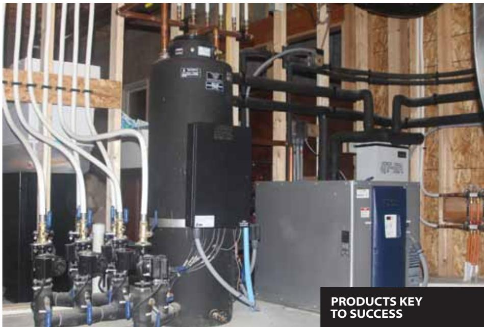
Above right, is the Envision water-to-water heat pump for radiant floor heat load. To its left is the B&D HSS non-pressurized buffer tank.
